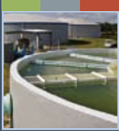
MUNICIPAL WASTE-WATER TREATMENT
